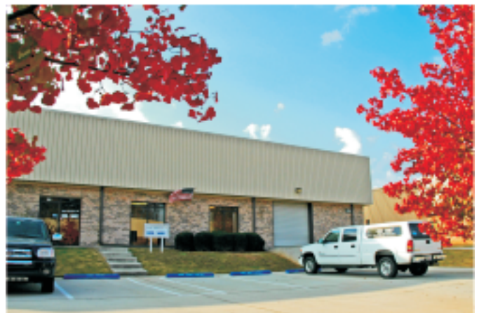
SHAHER HEADQUARTERS, STOCKBRIDGE, GA
